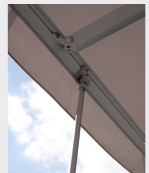
Telescopic support Stabilizes the awning when windy.
